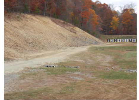
Bank cut back to facilitate roadway and #1 shooting position.
